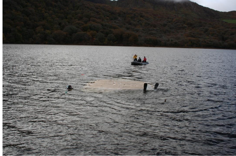
Laying Jute Matting in Deeper Water (to 7 metres) December 2016
