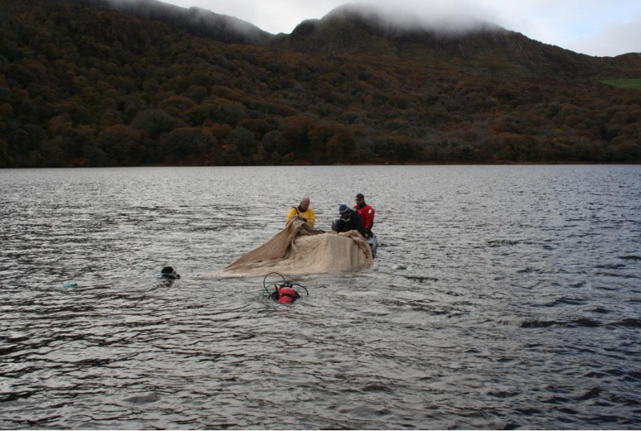
Laying Jute Matting in Deeper Water (to 7 metres) December 2016
