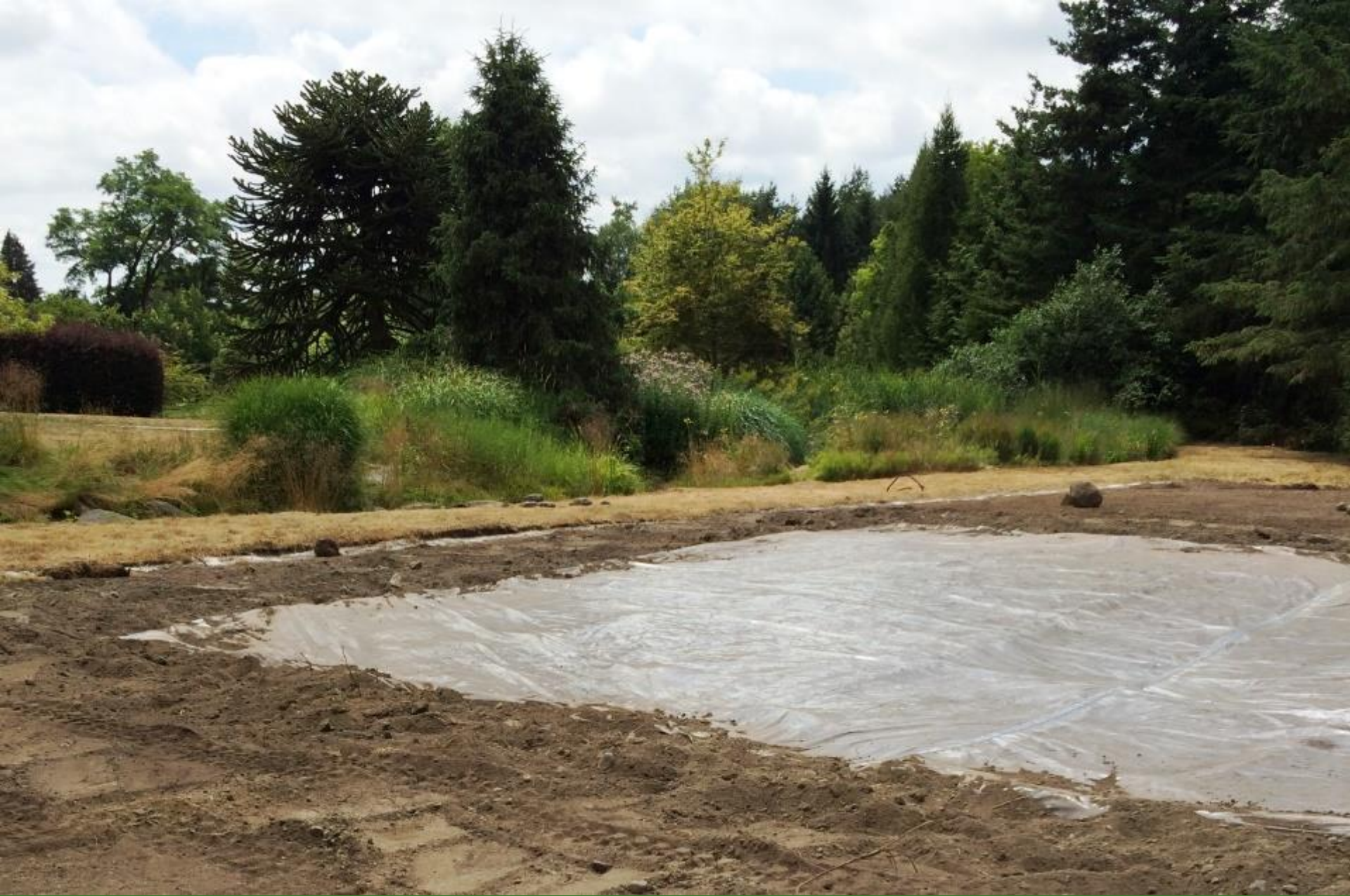
Filled in trench
